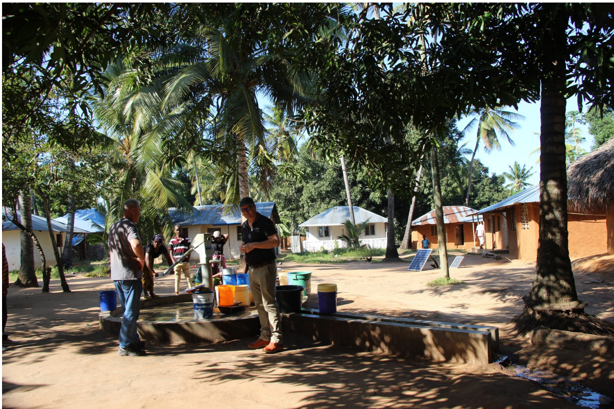
Infrastructure delivery — solar water tower project, Cabo Delgado.
