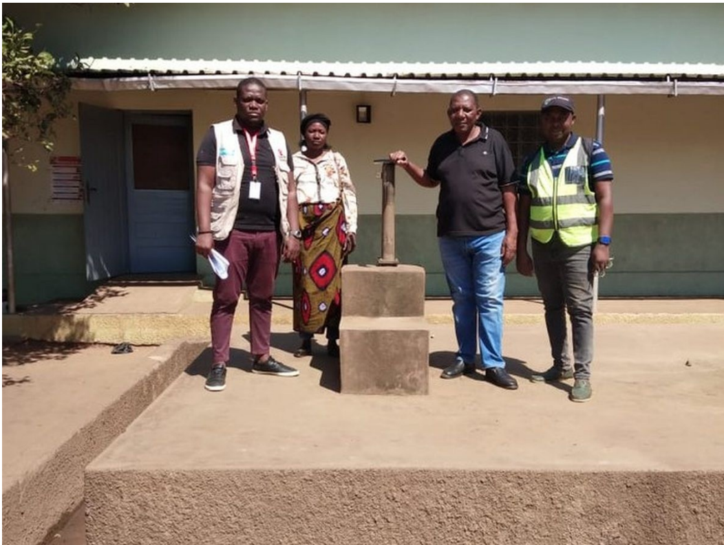
Community members at a rehabilitated Afridev handpump borehole in Chiúre district, southern Cabo Delgado.
