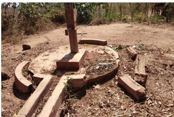
Before and after: a borehole with a cracked apron and failed pump (left), restored to full working order with a rebuilt, accessible surround (right).
