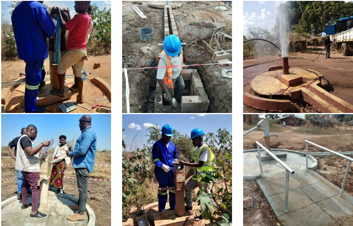
Top row: replacing worn Afridev pump components, rebuilding the drainage and headworks, and flushing the borehole until the water runs clean. Bottom row: inspecting and testing the pump, operating it with the community, and the finished, accessible water point.
