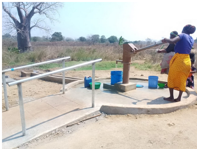
An ALPS handpump with an accessibility ramp and handrails, designed so that everyone in the community, including older people and people with disabilities, can collect water safely.
