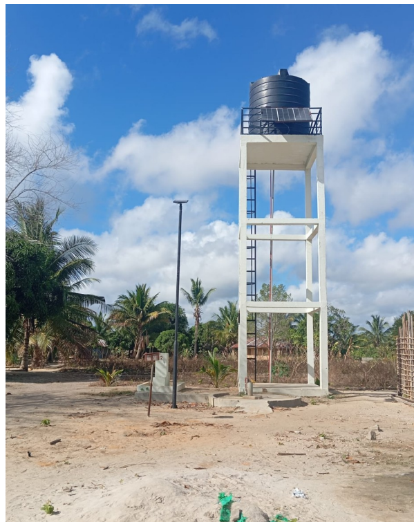
A solar-powered water tower delivered by ALPS. Reliable, low-cost water at the heart of the community.
